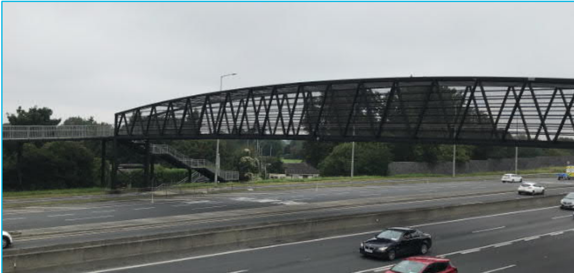
Photo 3 – Existing Liffey Valley Footbridge (east of proposed bridge location)
