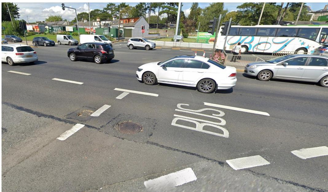
Figure 7-7 Good Road Pavement Condition on Chapelizod bypass, Palmerstown – (but with some damage around utility chamber covers) ©2020 Google Maps
