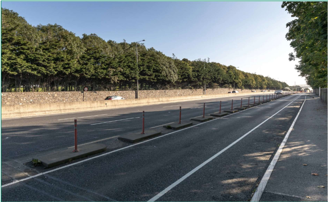
Figure 2.1.8: View 3 from the west – as existing
