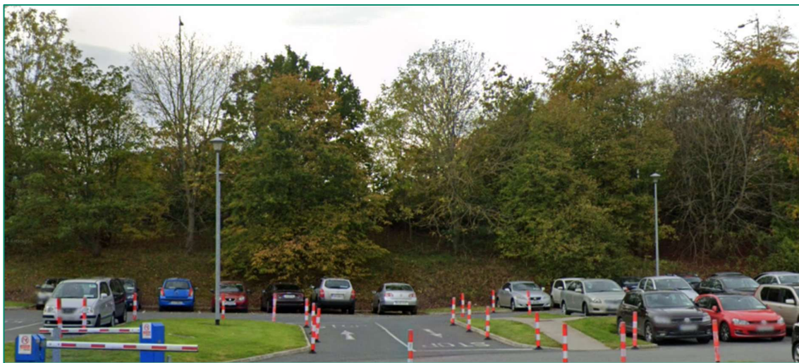
Figure 2.2.11: Existing Hermitage Medical Clinic Car Park and Side Slope to N4 (Image Source: Google)
