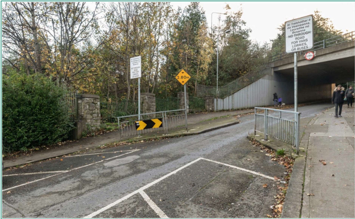
Figure 2.3.8: View from the north – as existing
