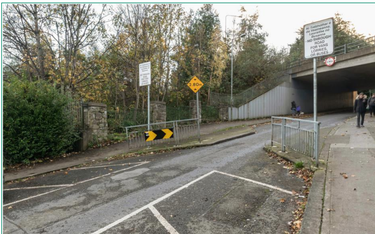
Figure 2.2.8: View from the north – as existing
