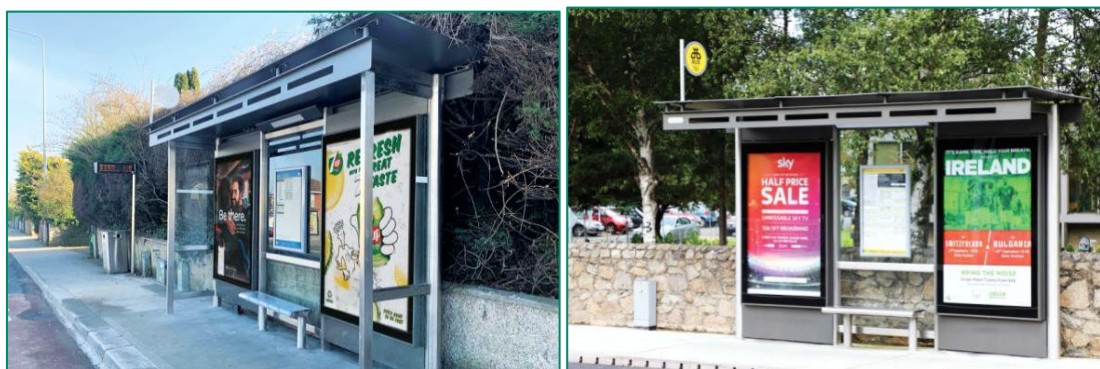
Figure 2.3.5.24: Example of a 3-Bay Reliance Cantilever shelter with a narrow roof configuration with and without half end
