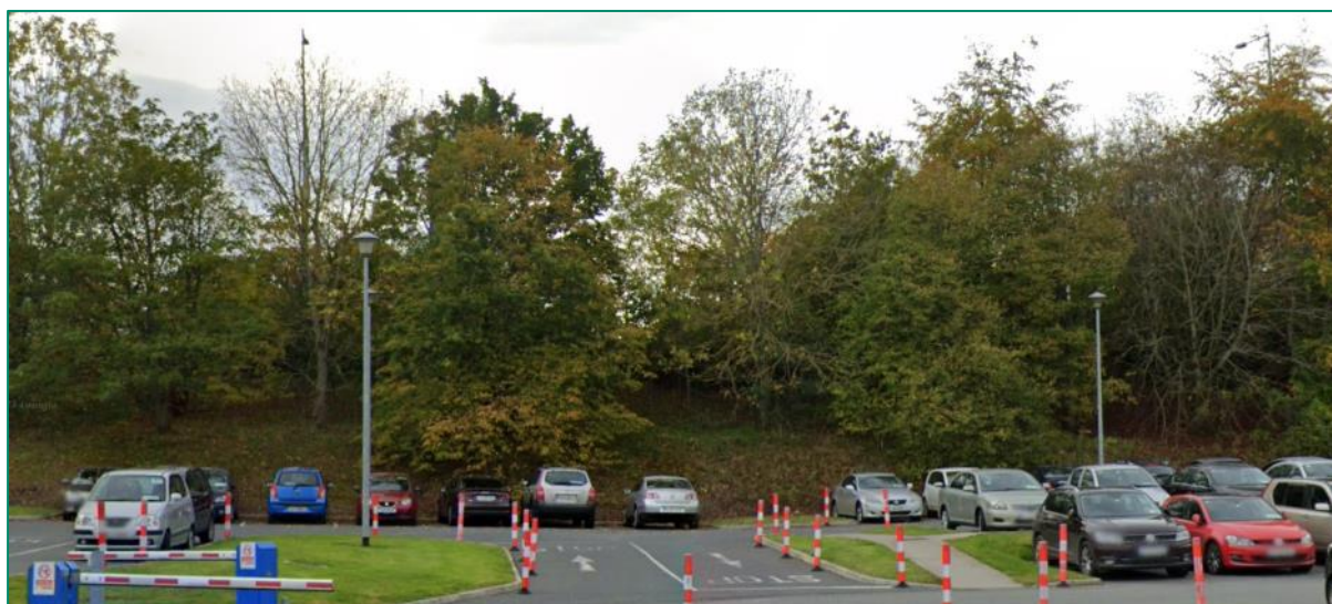
Figure 2.4.3.11: Existing Hermitage Medical Clinic Car Park and Side Slope to N4 (Image Source: Google)
